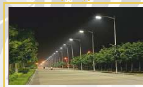
ELECTRIC LINE WITH STREET LIGHT
