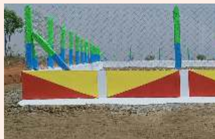
Open Space Wall & Net Compound
